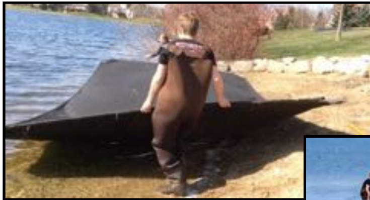
Carry from the 12-foot ends. (If alone, pull from a 12-foot end.)
